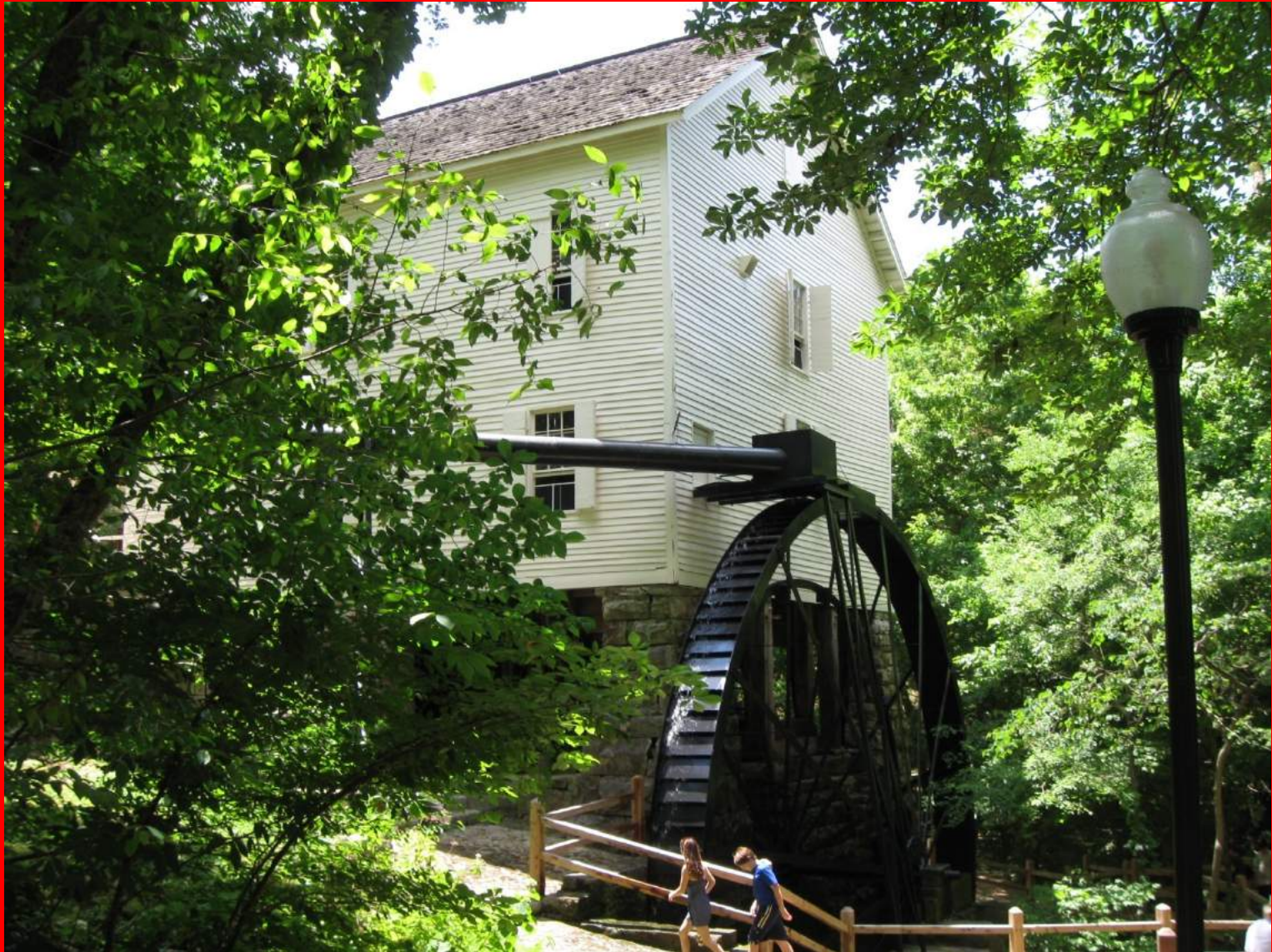
This is the Brown-Lanier Mill located near Mill Springs, Kentucky, near the Cumberland River. It is still an active mill. This image was taken by Robert Housch on Saturday, June 5, 2009.
