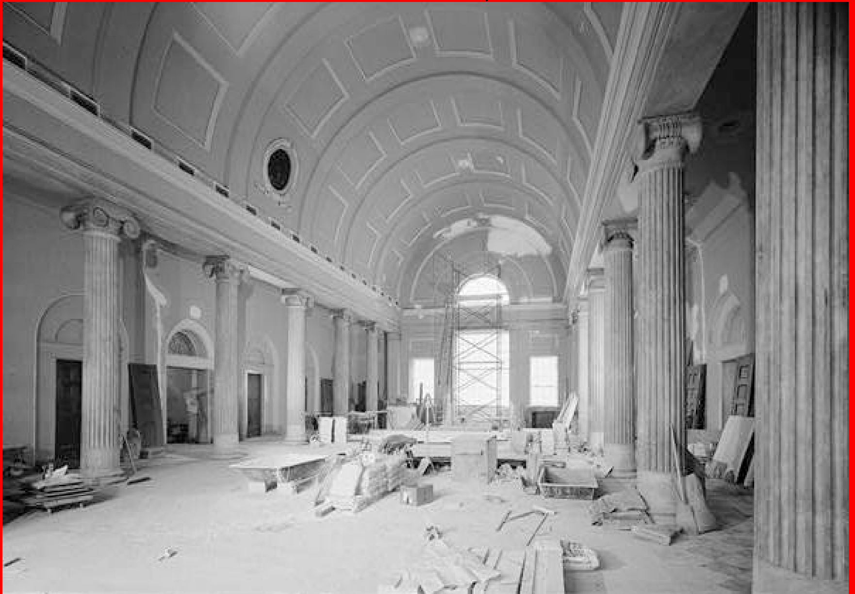
The Great Hall of the Second Bank of the United States in Philadelphia. This image was taken during renovation work by the National Park Service. This image is courtesy of the Library of Congress.
