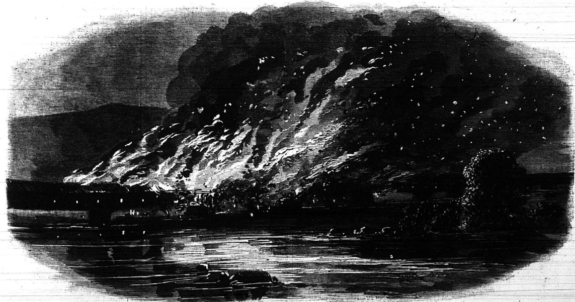
THE INVASION OF THE NORTH—DESTRUCTION OF THE BRIDGE OVER THE SUSQUEHANNA, AT COLUMBIA, PA.—SKETCHED BY A CORRESPONDENT.—[SEE PAGE 453.]
